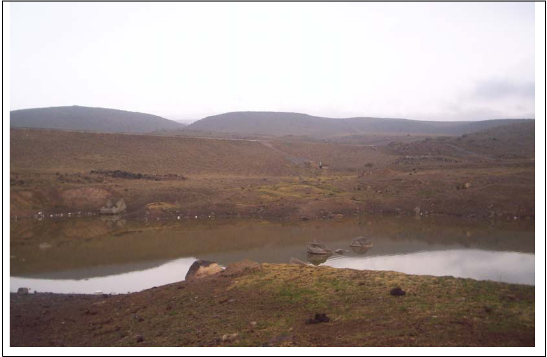
Fig. 2 View of downstream area of Kosh dam
